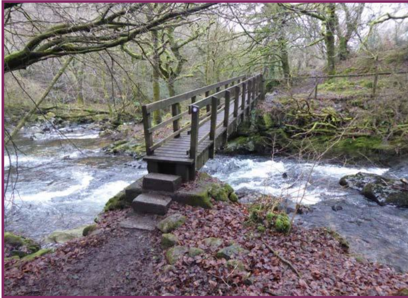
Tarka Bridge, Belstone Cleave
